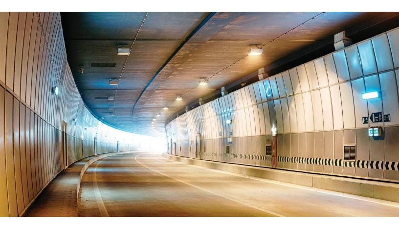
Installation ease was another key factor contributing to the project's overall success. "Compared to other materials, CeramicSteel panels are lighter and the surface is flexible enough to fit the tunnel's curve," Senyuk says.
